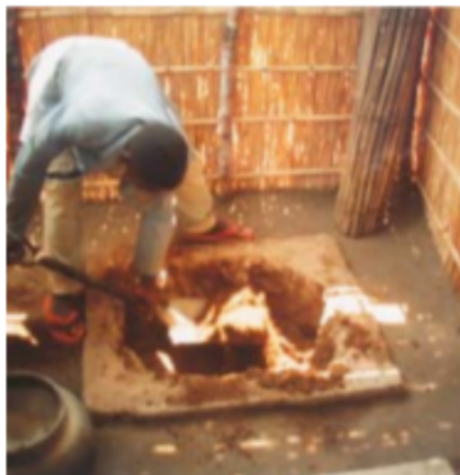
excavating the humus from the pit
